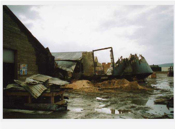
Aftermath of the 2002 fire
