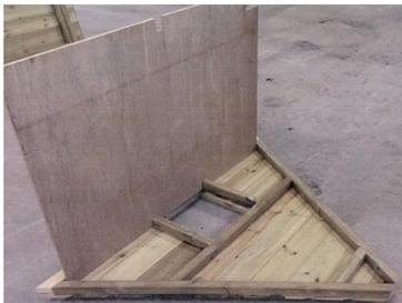
Starting with the apex panel (with doorway), slide the floor into position and fix with 2x 40mm screws. The floor has two slots cut out to fit over the doorway.
