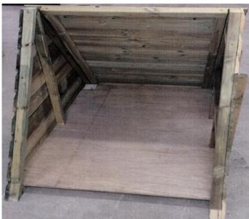
Next slot the front hinged door panel into position, on the opposite side to the back panel and secure with 4x 90mm screws.
