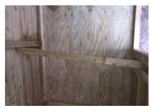
Fix the perch using 2x 90mm screws to the back and the front panel.
