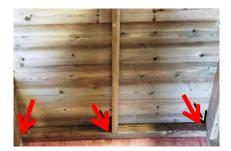
Fix the back panel to the base using 3x 90mm screws.
