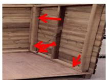
Screw side panel to base and back panel using 4x 90mm screws.
