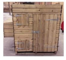
Screw the front panel on using 4x 90mm screws.
