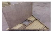
Start with apex panel (with doorway). Slide floor into position and fix using 2x 40mm screws. (The floor has two slots cut-out to fit over doorway).
