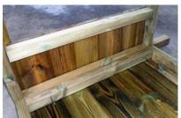
Fix the three base supports into the bottom of the kennel using 6x 60mm screws and place the ply base section into position.
