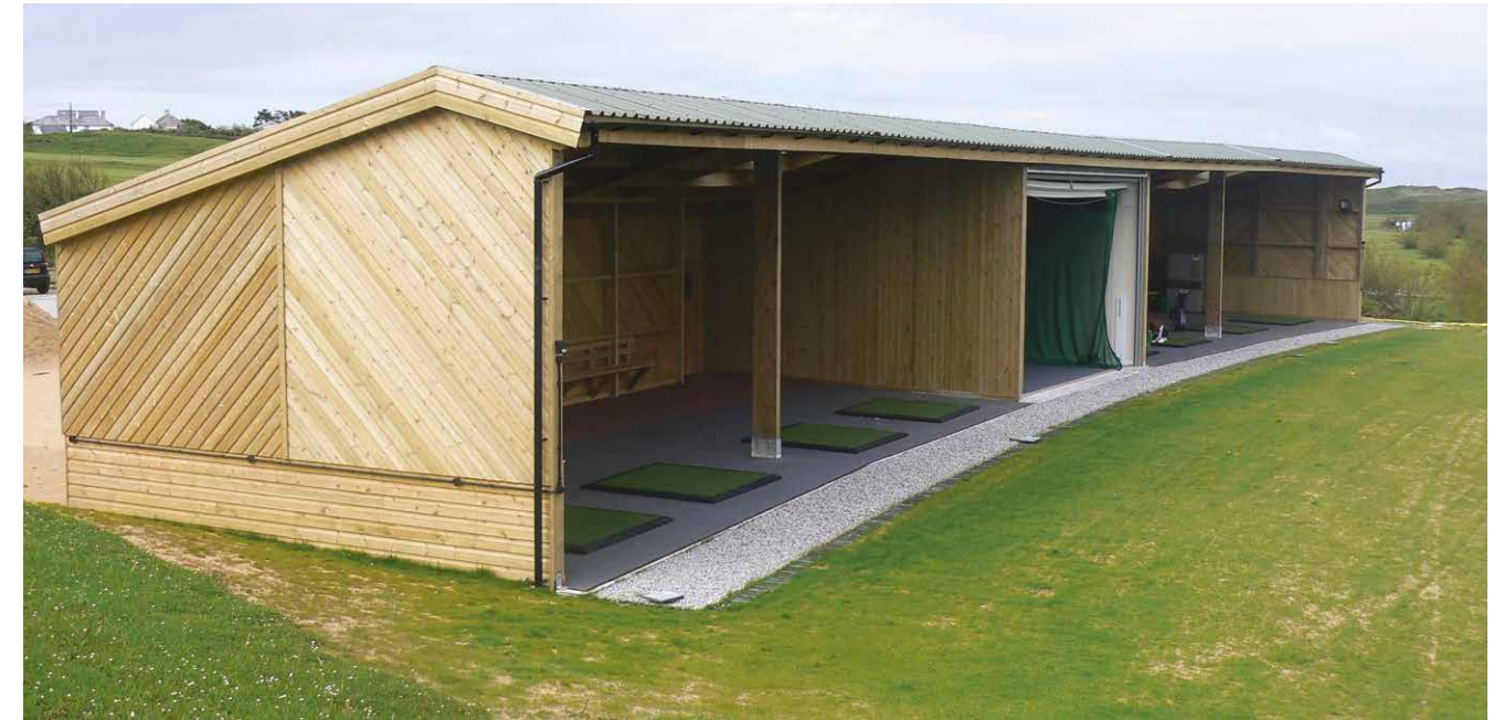
Photo above: Monopitch timber framed structure with an oversail feature at the front.
