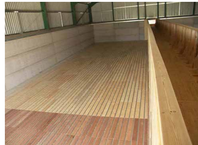
View of a Lingward composite drying floor from the main air duct
