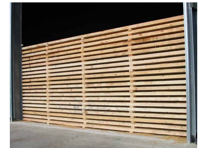
Doorway infill boards
