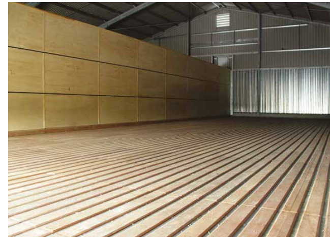
Lingward drying floor and main air duct for 3.66m storage.
