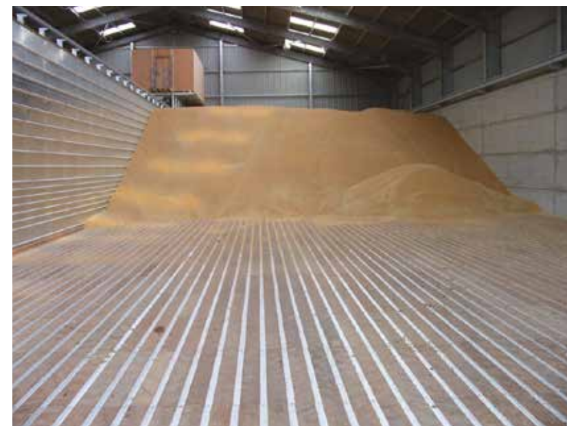
Photograph above: Drying floor with steel air duct Top right: Main air duct
