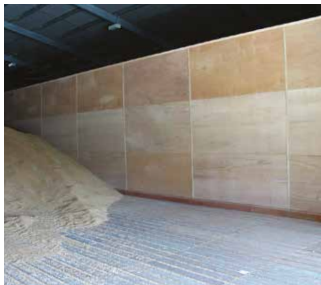
Drying floor with timber air duct
