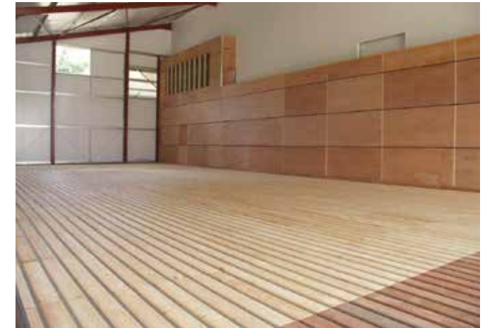
Vegetable store with ventilation and refrigeration fitted to a Lingward main air duct and floor.
