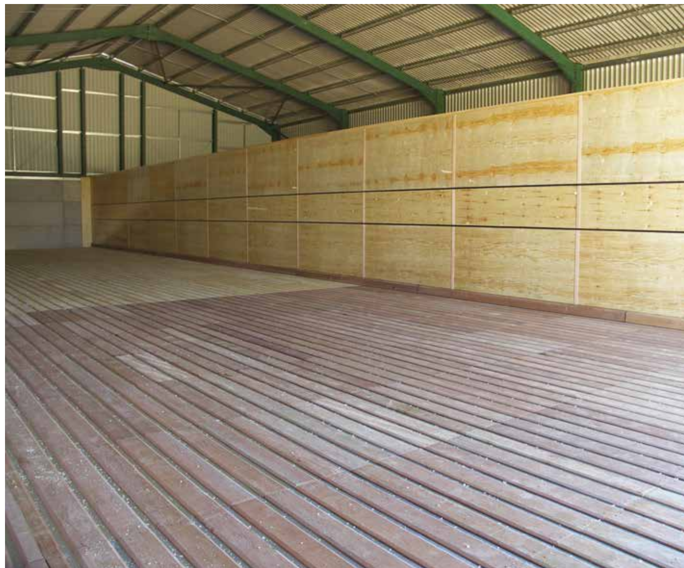
A composite hard and softwood Lingward floor fitted with a Lingward main air duct.
