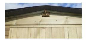
7. Nail the felt around the outside of the roof every 100mm.
