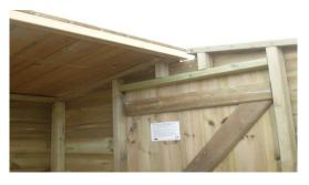
3. Place one roof panel on to the top of the shed. The batten will fit into a central recess on the front and rear panels. Repeat for the other panel. Then screw into place using seven screws into each roof panel. Once the roof is screwed into place, fix the panels to the floor section. Use three screws for each side panel and two screws each for the front and back panels.
